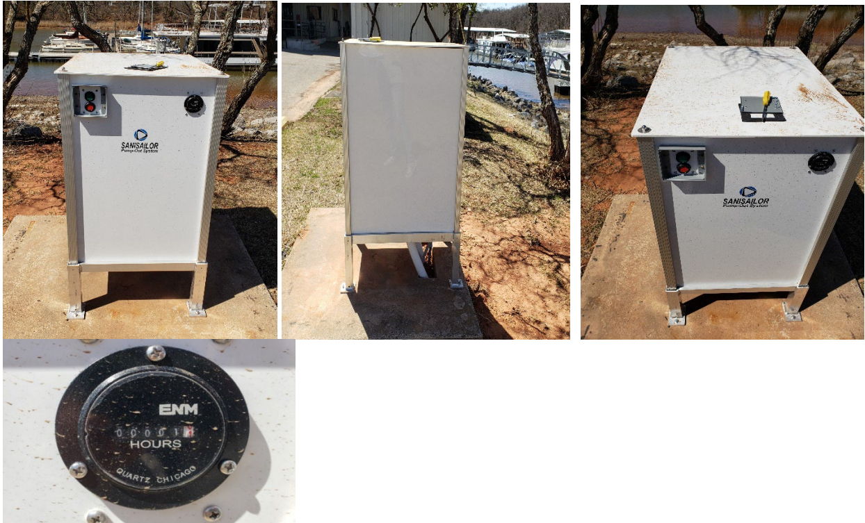
Photo Series #3. Calypso Cove Marina on Lake Thunderbird. April 1, 2022. Brand new lift station on shore by marina dock.
