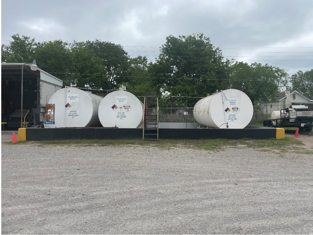
Figure 6: Tank Farm with Secondary Containment
