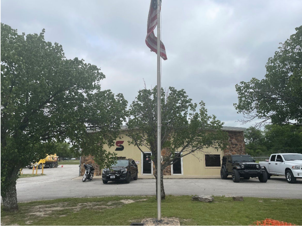
Figure 1: Main Office Building
