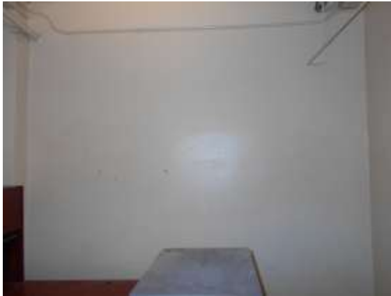
Photo #3: Room #15 Wall A Bldg 1919
