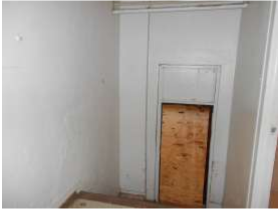
Photo #1: Room #7 Bldg 1919
