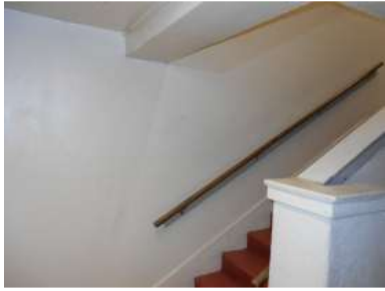
Photo #4: West Stairway Wall Bldg 1919
