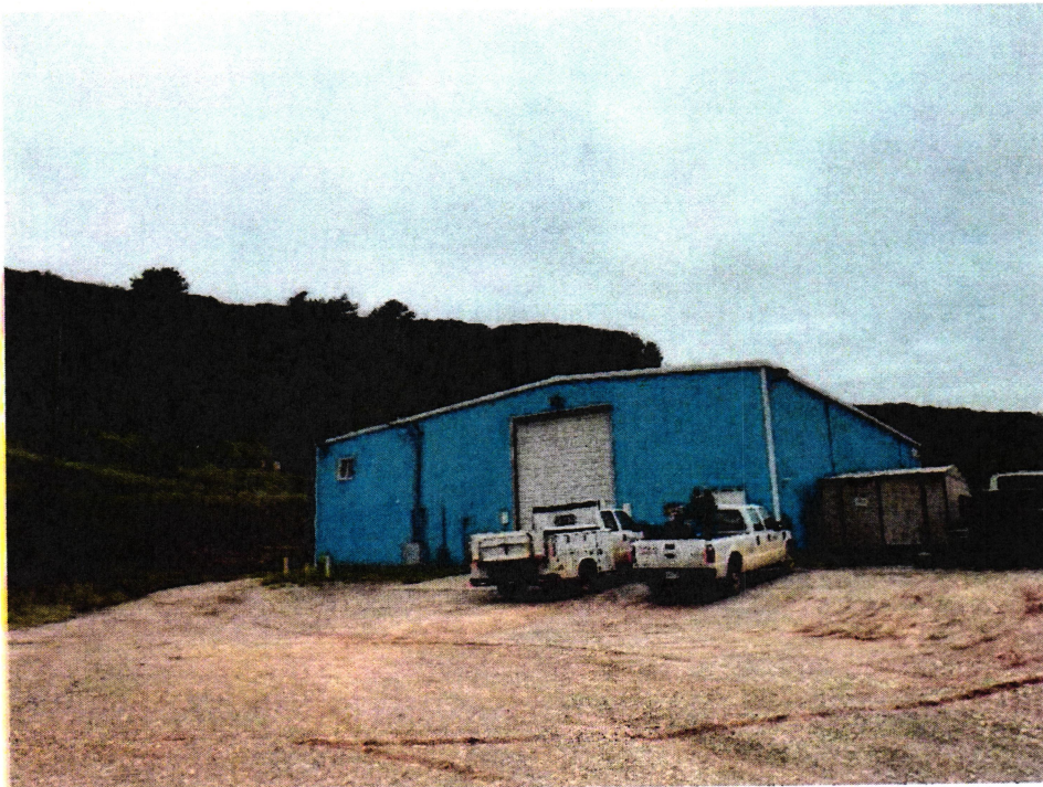
Entrance to General Maintenance Building
