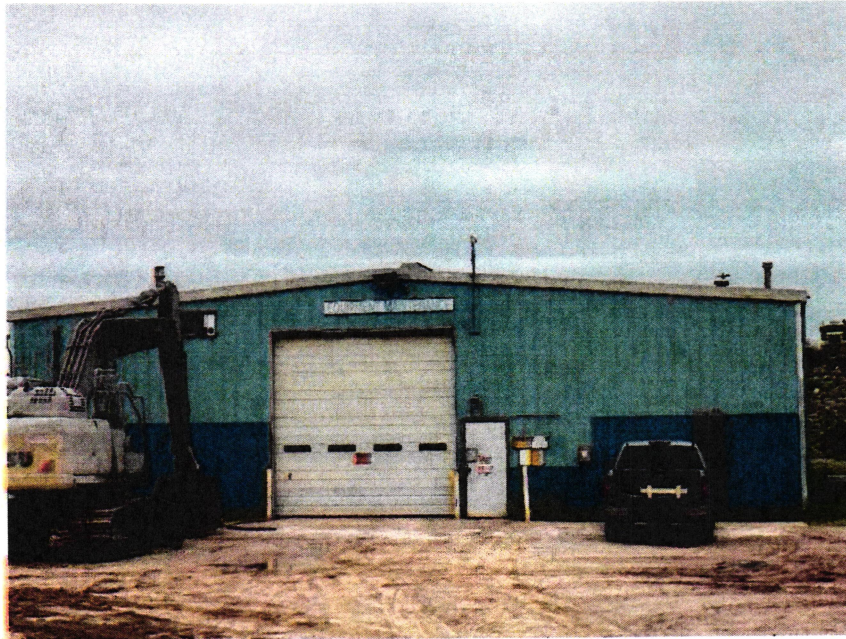
Equipment Maintenance Building
