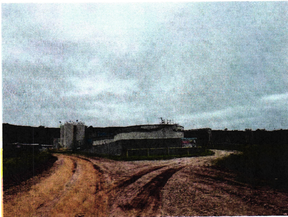
EF Tank Storage Area
