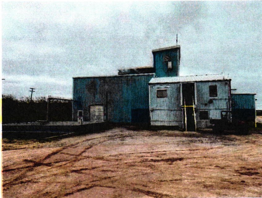
Wastewater Final Treatment Building
