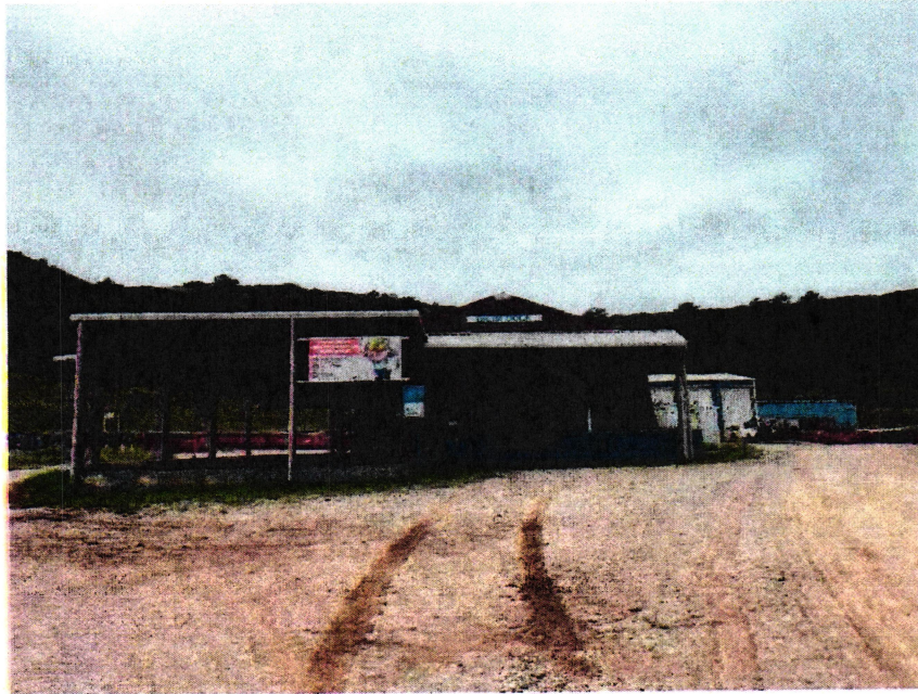
Drum Dock Building
