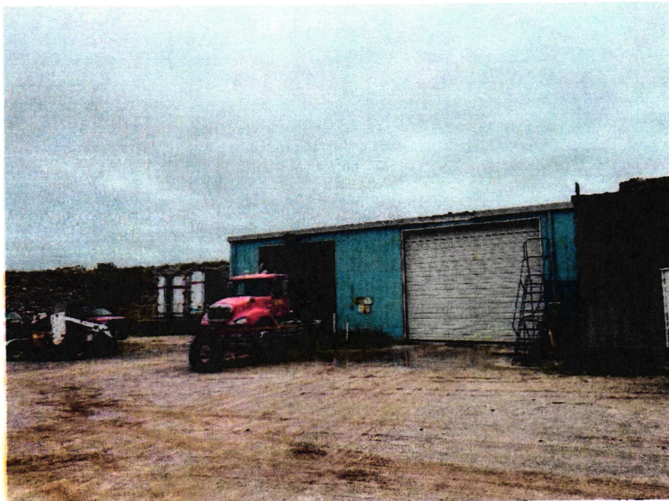
West side of Equipment Maintenance building
