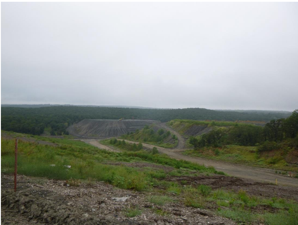
Figure 6. View of backfill from the current landfill in APE; view to northwest.
