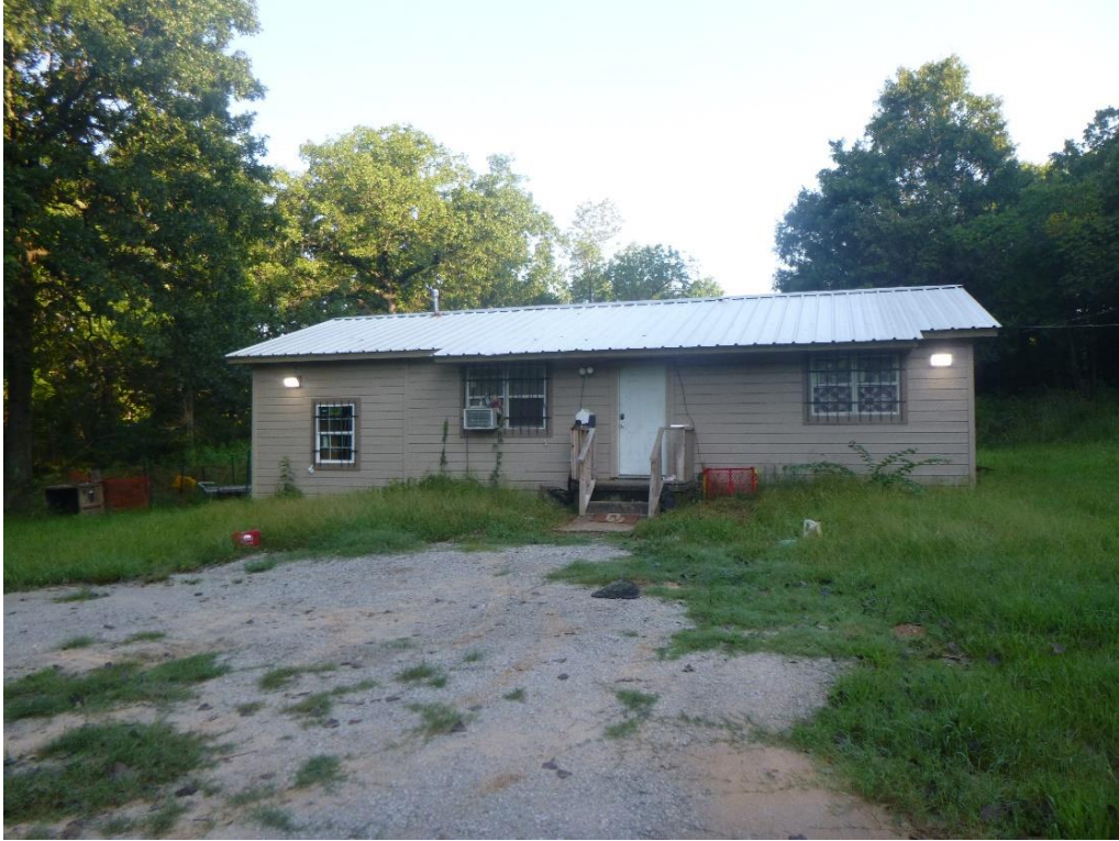
Figure 17. Building 1A; facing west.
